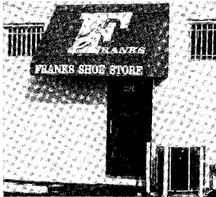
A new look for Frank's Shoe Store who took advantage of the TIF Program (front and back of building).
